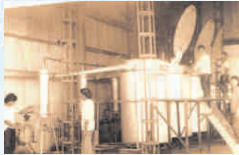
Distillation plant in Yaongyimsen
