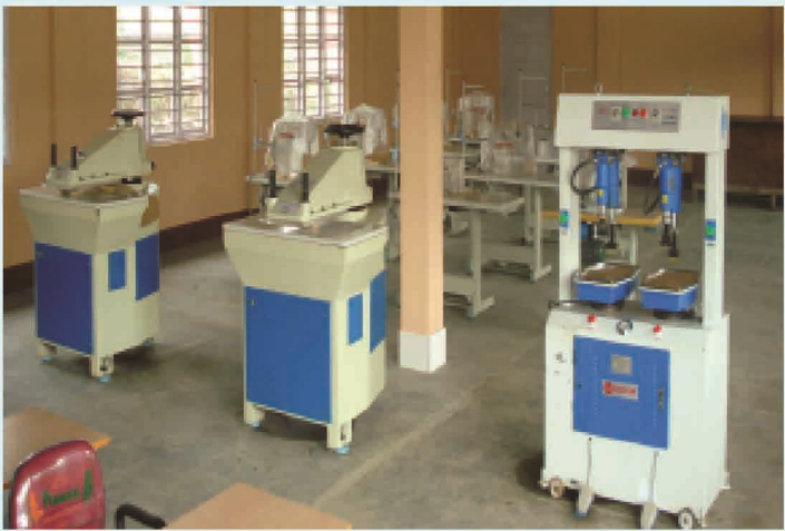
Hydraulic clicking and pneumatic sole attaching machines at the Substation
