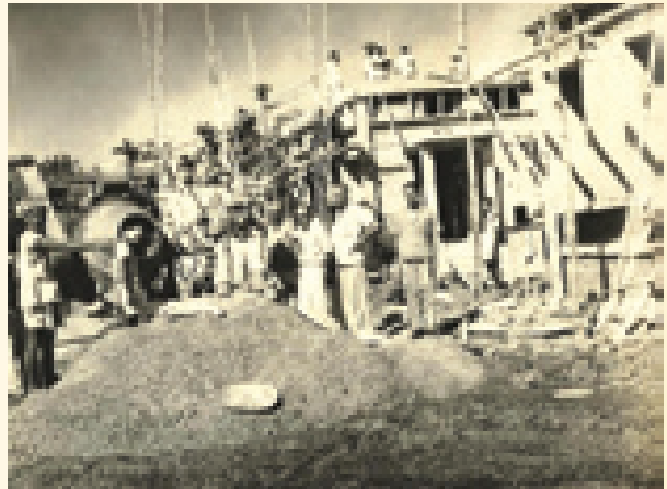
The initiation of the construction of laboratory Administrative building
