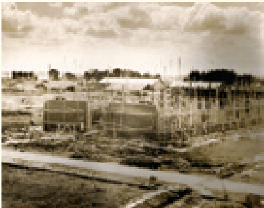
The construction is in full swing
